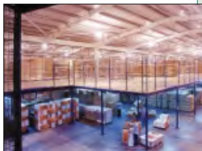
• Steel structural work incorporating a mezzanine floor
