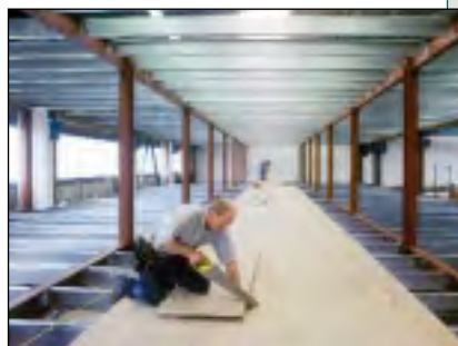
• Office and floor construction
