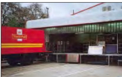
• Loading dock installation for the Royal Mail
